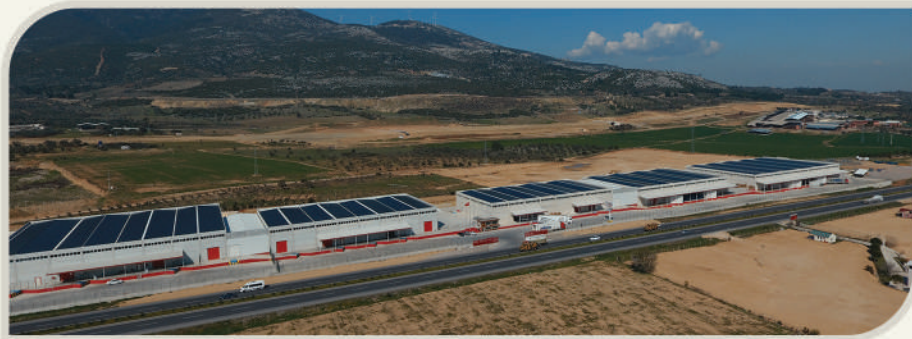
Oto Irmak 2.2 mW Roof Solar Power Plant > İzmir - Türkiye
