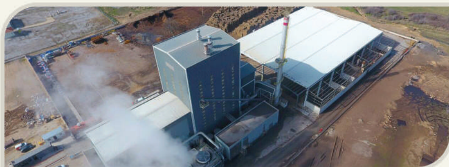
Zeus Energy Biomass Energy Plant > Kırklareli - Türkiye
